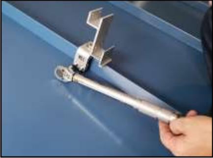
**Once all RoofClamp/RC-2B assemblies in the bar section are installed, torque all set screws to 90 inch/lbs. while applying downward pressure to the bar.**
